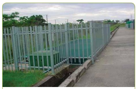
Water savings project, FNB Fort Jackson – FNB's injection moulding factory at Fort Jackson uses rainwater for cooling moulds and machines. In 2011 municipal water was only accessed for two days. The ultimate goal is to become completely independent of the municipal water supply by adding a closed loop refrigeration system, storage capacity and linking to the wastewater system.
